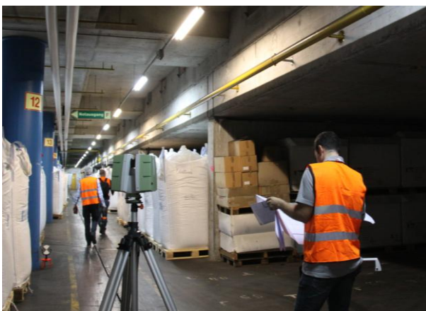
Scanning process. With the red circle is emphasized the usage of portable black and white targets in order to constrain the scans
